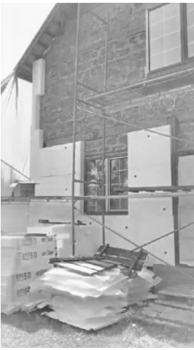
They began to put insulation panels outside and inside of the walls.
